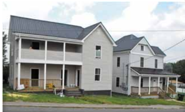
Mary Street renovations, Bristol, Virginia
