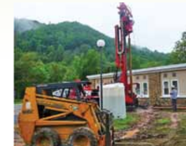
Above: Vertical wells were dug for the geothermal heating/cooling system.
